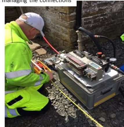
Blowing fibre & managing the connections
