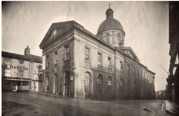
Pre 1925 view of west end of Market House Image courtesy of Penlee House Gallery & Museum, Penzance
