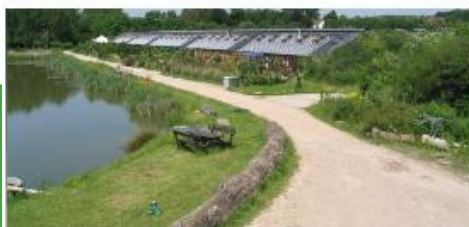
Hockerton Housing Project
