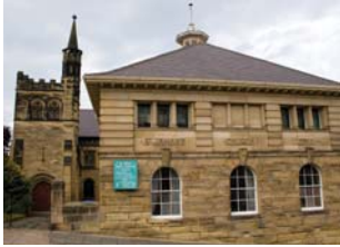
St James's church hall, now converted into 9 affordable homes
